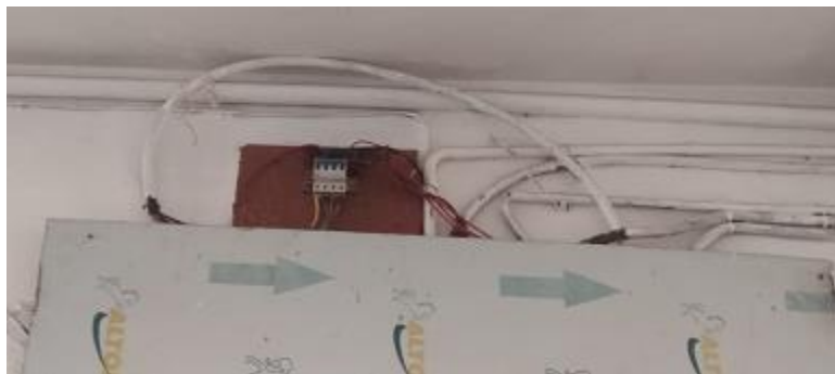
In-accessible switchgear
