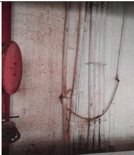
Old Conduit and Hanging wire
